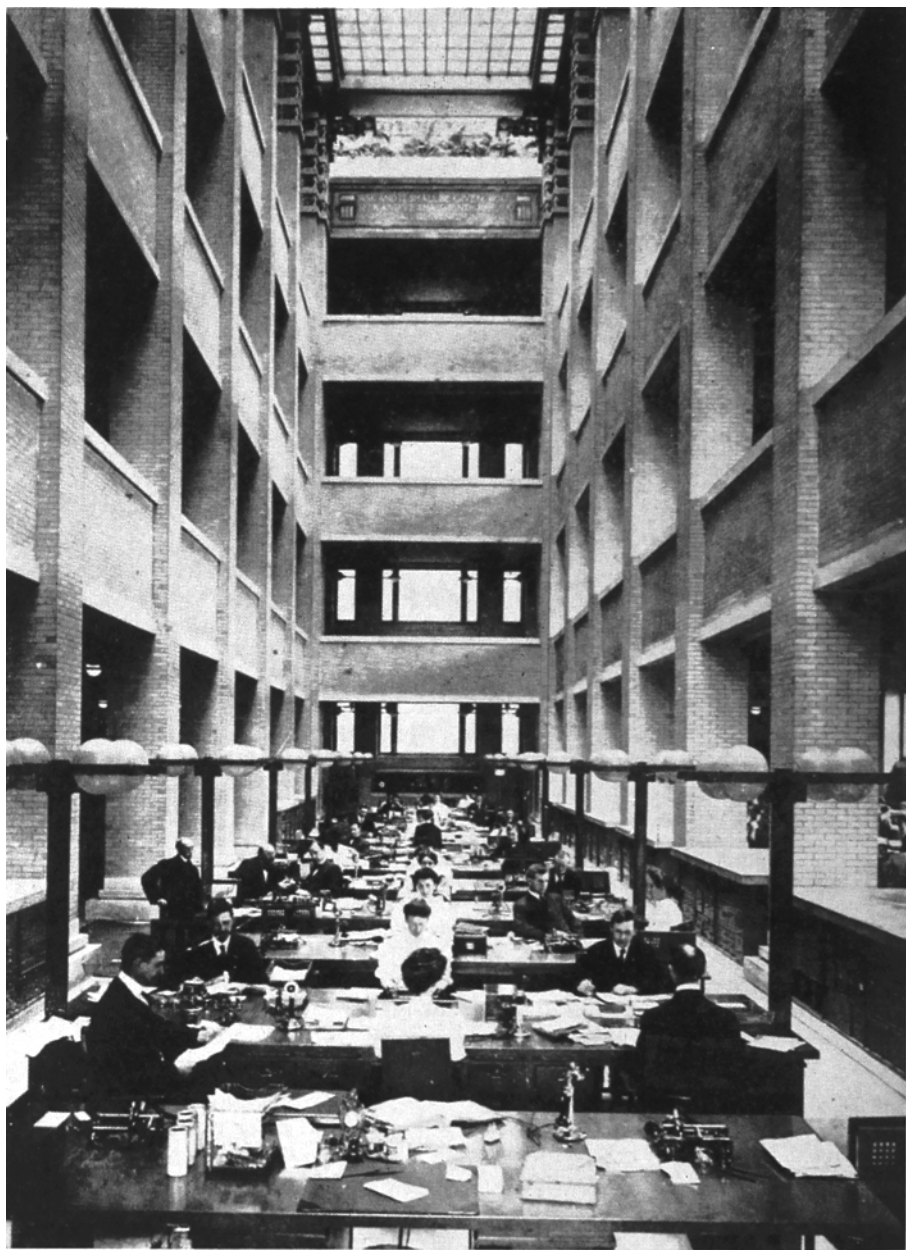
Fig. 8. F. L. Wright: Interior of Larkin Building, Buffalo, N.Y., 1904.
